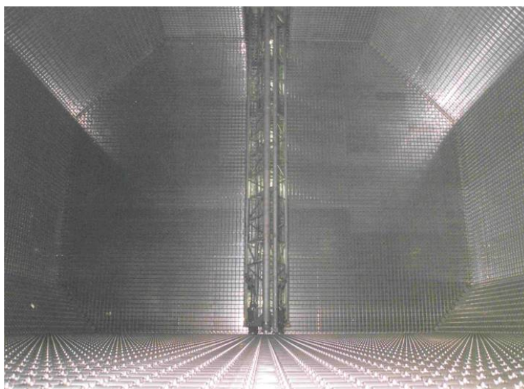
Figure 1.7: Membrane: Technigaz type Mk III
